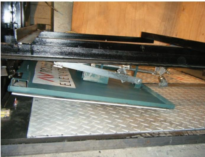
gear mechanism/UCMP of the elevator and operates using an overspeed governor (OSG), rope activation or a solenoid, which, for example, activates an existing anti-creeping/UCMP device.
